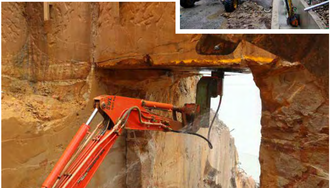
🕒 Cutting sandstone horizontally with Echidna D3 diamond rocksaw. (Sydney, Australia)
